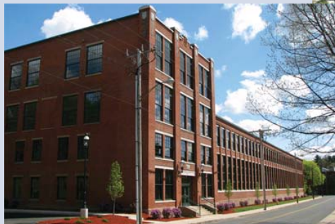
photo: Crosskey Architects, LLC
