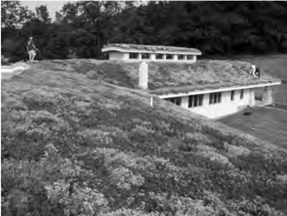
An extensive green roof by Charlie Miller, Roofscapes, Inc., for the Chiropractic Life Expression Wellness Center in Sugar Loaf, Pennsylvania.
