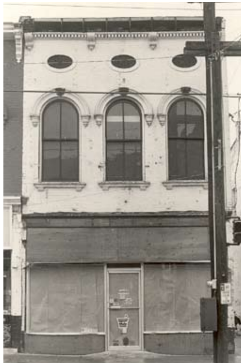
The storefront on this Victorian building prior to rehabilitation was a later replacement (left). During rehabilitation the storefront was removed and replaced with three residential-type openings that are incompatible with the building's retail character (right).
