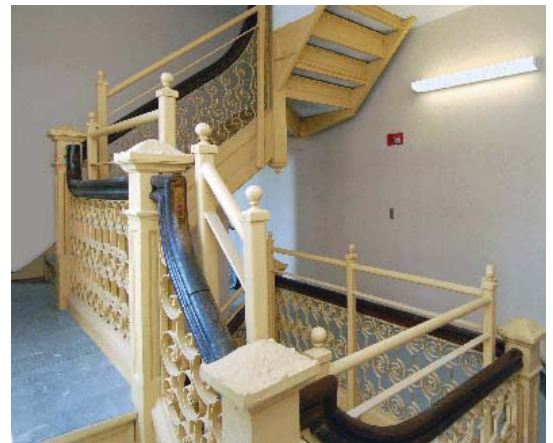
Right: Revised railing that better relates to historic design and meets the Standards.
