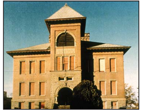
1901 school building prior to rehabilitation.
