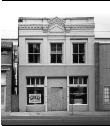
Commercial building prior to rehabilitation.
