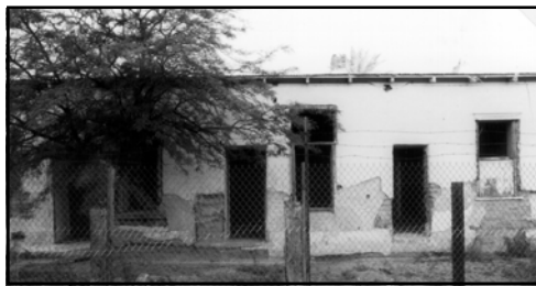
Adobe apartments prior to rehabilitation.
