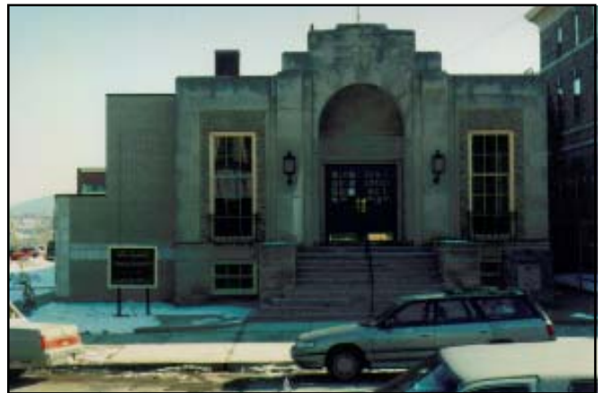
After rehabilitation. The addition is located very close to the facade and, as a result, is highly visible, altering the symmetrical balance of the historic facade.
