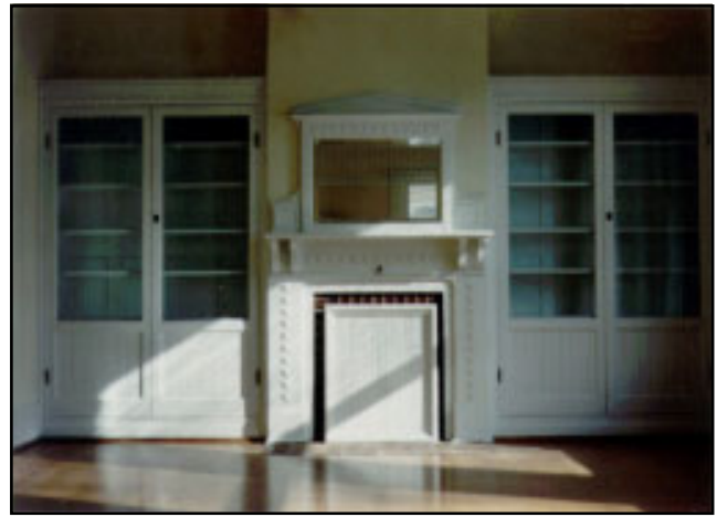
During rehabilitation most of the naturally-finished woodwork was painted white, resulting in a drastic change of character to this late-nineteenth century interior.
