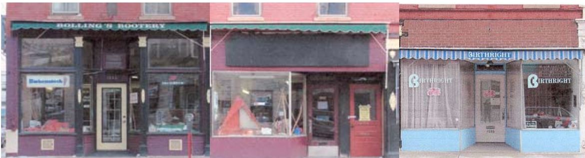
Details of existing storefronts prior to rehabilitation.
