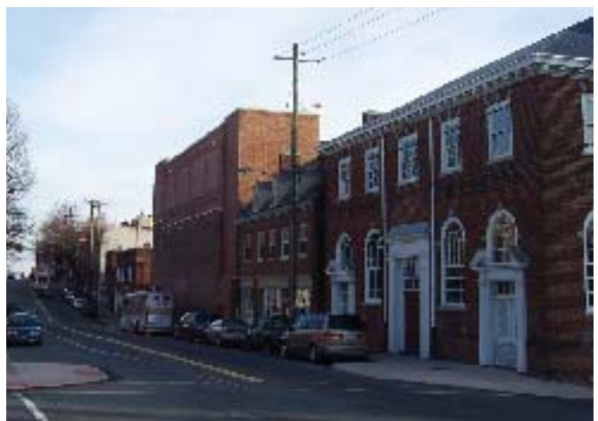
The new fly loft redesigned to meet the Standards is shown here after rehabilitation.
