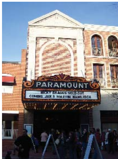
Left: Front of Colonial Revival-style movie house after rehabilitation. Due to the length of the building (a full block long), the added fly loft is only visible at the rear of the site.
