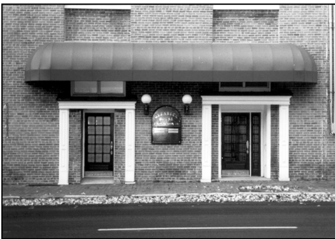
Side entrances with single continuous awning.
