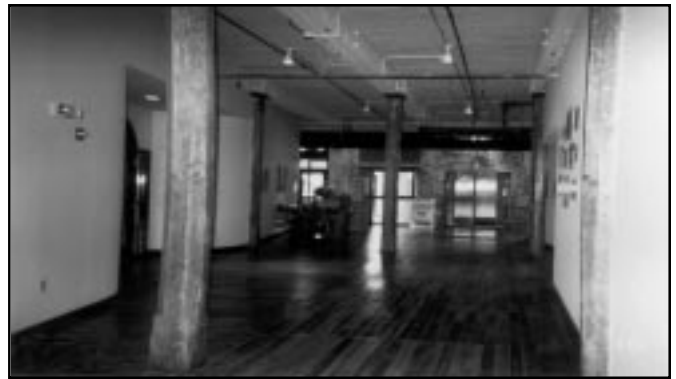
Interior after rehabilitation retains the exposed structure and finishes characteristic of the mill building with subdivision of the space for the new use.
