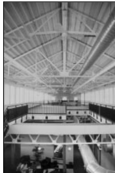
Interior following rehabilitation showing exposed latticed I-beams and metal trusses.
