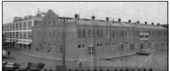
Tin can factory following rehabilitation.
