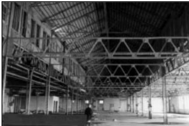
Second and third floor truss system before rehabilitation.
