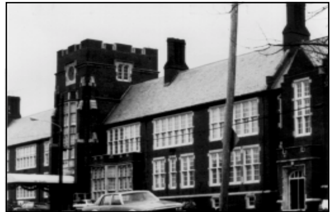
School after rehabilitation.
