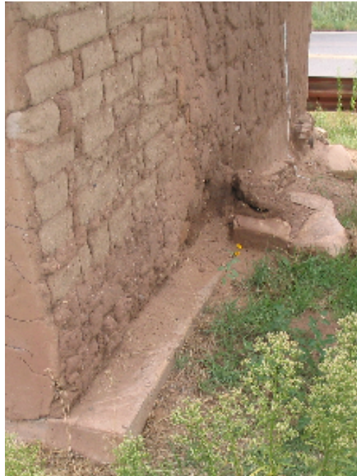
West wall showing 1983 concrete foundation
