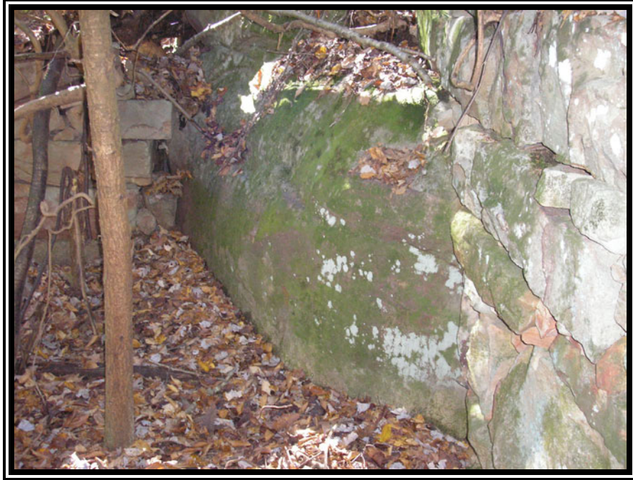
Figure 5.32. Large boulder incorporated into wall of possible mill at Carnifex Ferry.
