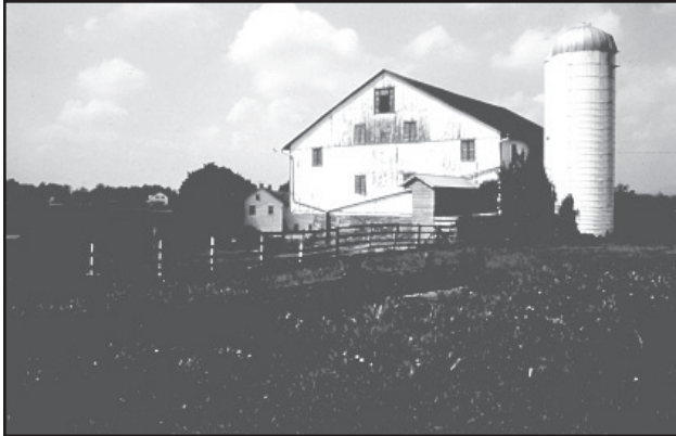
Figure 3.59. Farm #3 bank barn and silo, east facade, farmhouse in background, May 1969. (W. E. Dutton, EISE NHS files)
