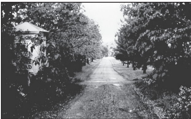
Figure 3.45. Guardhouse on Farm #2 entry drive, vegetation overtaking structure, cattle guard across drive in middle of photo, view toward west, May 1969. (W. E. Dutton, EISE NHS files)
