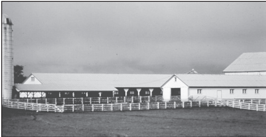
Figure 3.37. Maternity shed, loafing shed, silo, and corrals on Farm #2, view toward southwest, May 1969. (W. E. Dutton, EISE NHS files)
