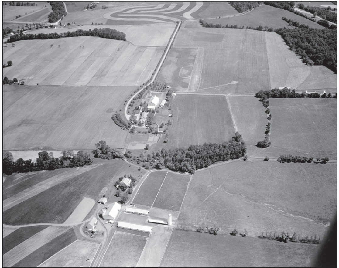
Figure 3.10. Aerial view of Farms #1, #2, and #3 from the south, contour stripping evident in the fields, 22 June 1964. (Lane Studio, EISE NHS files, #2973)
