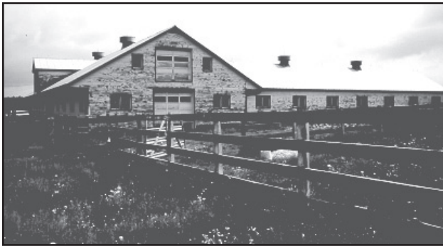
Figure 3.43. Show Barn and corrals, south facade, May 1969. (W. E. Dutton, EISE NHS files)
