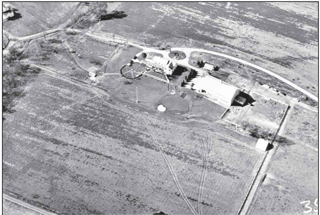
Figure 3.14. Circulation improvements during the Eisenhower period soon after installation, paved entry road, gravel farm road to eastern fields in right of photo, Nevins Lane in lower left corner, access to Farm #2 in upper left still in use during construction on Farm #1, late fall 1955. (EISE NHS files, #3136)
