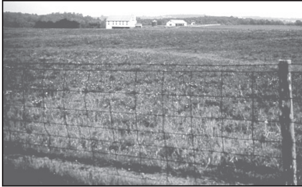
Figure 3.26. Post and wire fencing with barbed wire top, along Millerstown Road on Farm #3, view toward northwest, May 1969. (W. E. Dutton, EISE NHS files)
