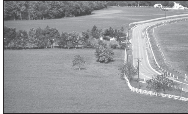
Figure 3.25. Cross-board wooden fencing along Millerstown Road on Farm #1 side, post and wire fencing on Farm #3 side, May 1969. (W. E. Dutton, EISE NHS files)
