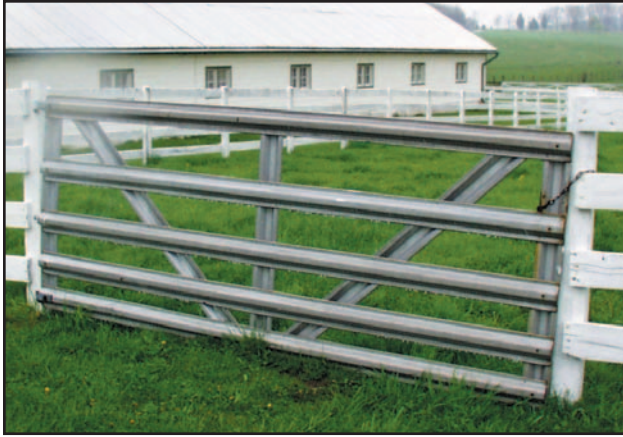
Figure 3.32. Steel farm gate. (Photo by OCLP, 2002)
