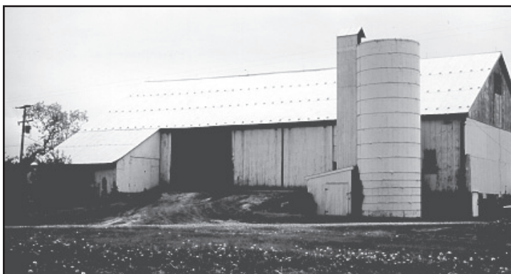
Figure 3.38. Farm #2 bank barn, west facade, May 1969. (W. E. Dutton, EISE NHS files)
