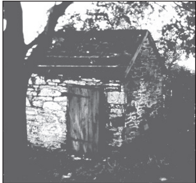
Figure 3.58. Farm #3 smokehouse, east facade, May 1969. (W. E. Dutton, EISE NHS files)
