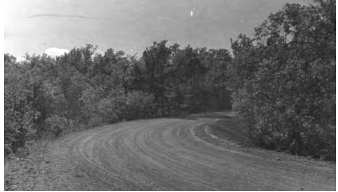
Figure 4-7. Completion of fine grading on Perimeter Road near Buffalo Springs, circa 1935.
