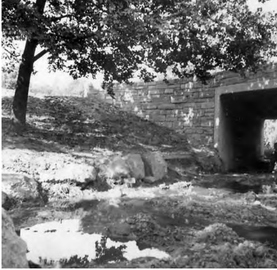
Figure 4-12. Fine grading and rip-rap by CCC crews at the Traver-tine Creek Bridge, circa 1934.
