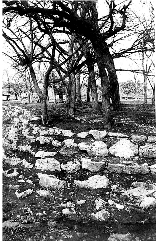
Figure 4-53. Detail of revetment wall construction, 1935. Note comfort station in left hand side of photograph.
