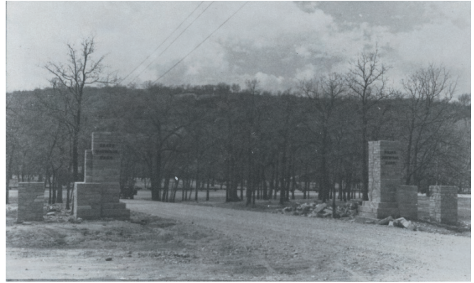
Figure 4-22. Completed set of entry piers at 12 th Street and Lindsay Avenue, 1935. Note that iron lettering is located on both large piers.
