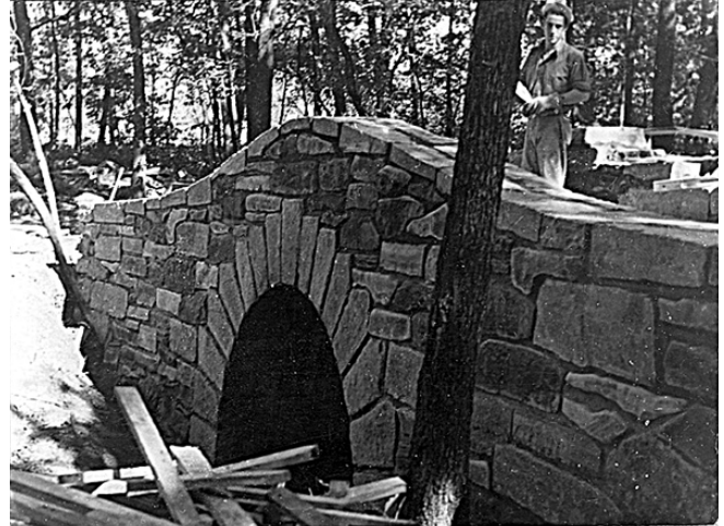
Figure 4-16. Construction of curved stone arch footbridge at Buffalo Springs, 1935.
