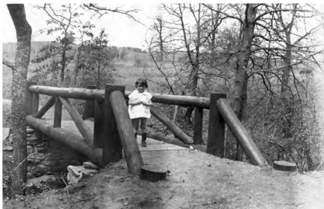
Figure 4-14. Typical peeled log trail bridge, circa 1935.
