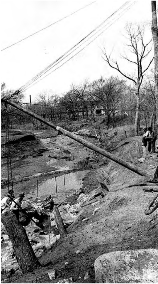
Figure 4-52. Placement of rip-rap using winches at the Flower Park revetment wall, 1934.
