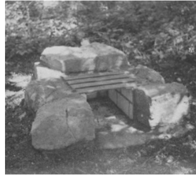
Figure 4-83. Stone masonry fireplace at Cold Springs Campground, circa 1935.
