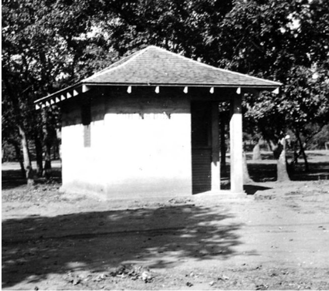
Figure 4-19. New concrete stucco comfort station at Bromide Springs, 1932.
