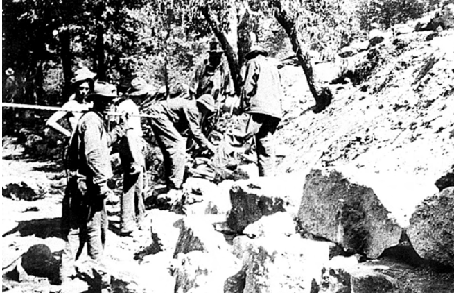
Figure 4-9. Laying rip-rap wall at Horner's Bluff, circa 1934.
