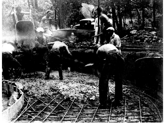
Figure 4-98. Buffalo Spring under construction, 1934, showing concrete reinforcing.
