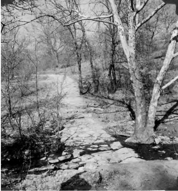
Figure 4-15. Typical stepping stone trail crossing “near Cold Springs Campground,” on Buffalo Springs trail, circa 1935.
