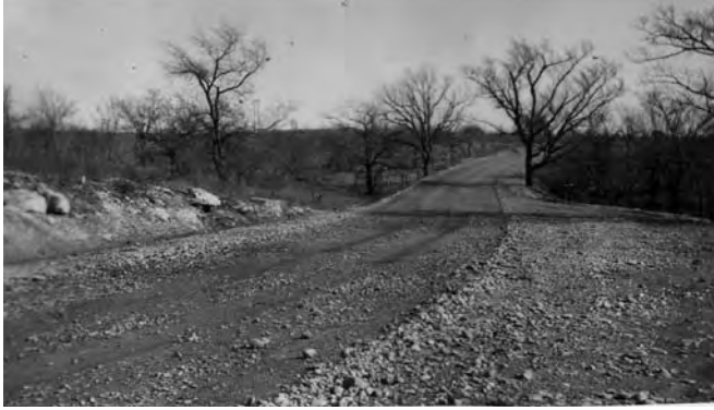
Figure 4-6. Construction of the perimeter road near Buffalo Springs road culvert, circa 1934. Picture shows completion of rough grading. Note the parking lot on the right.
