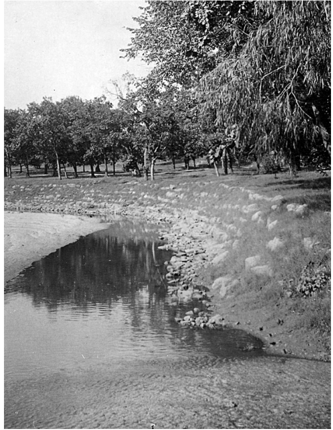
Figure 4-54. Completed revetment wall in Flower Park, 1935.
