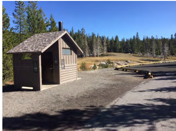
An accessible route is needed to the new vault toilet
