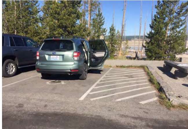
Accessible parking space and access aisle (no curb cut)
