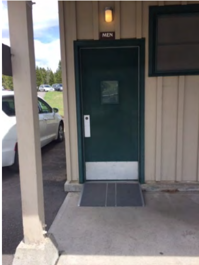
Marina comfort station (men's)
