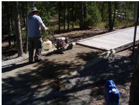
Repairing transition from trail to boardwalk
