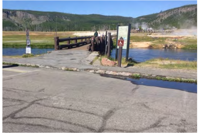
Biscuit Basin accessible parking space
