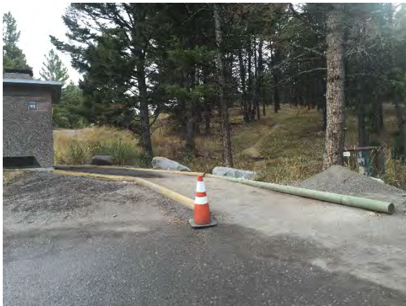
Upper Terraces vault toilet
