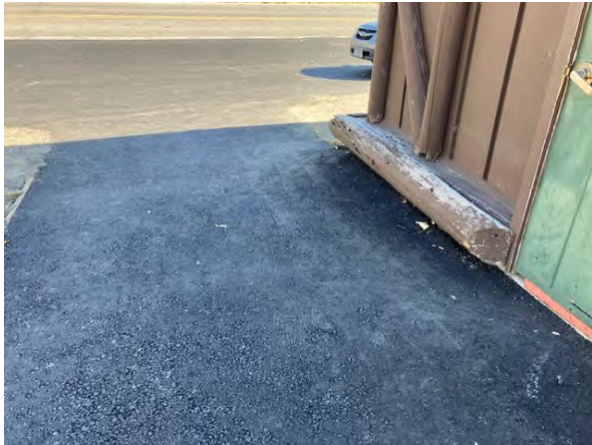
Accessible route to comfort station from parking area
