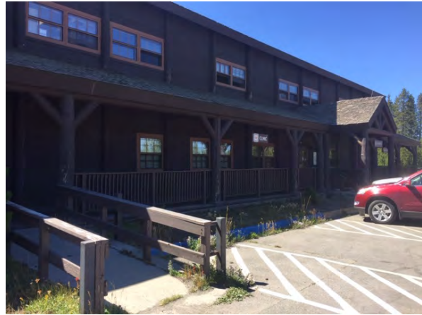
Ramp and parking at clinic
