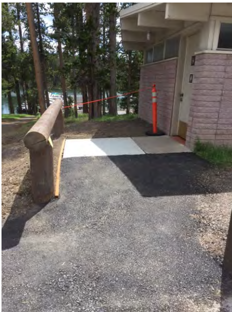
Bridge Bay picnic area comfort station (women's)
