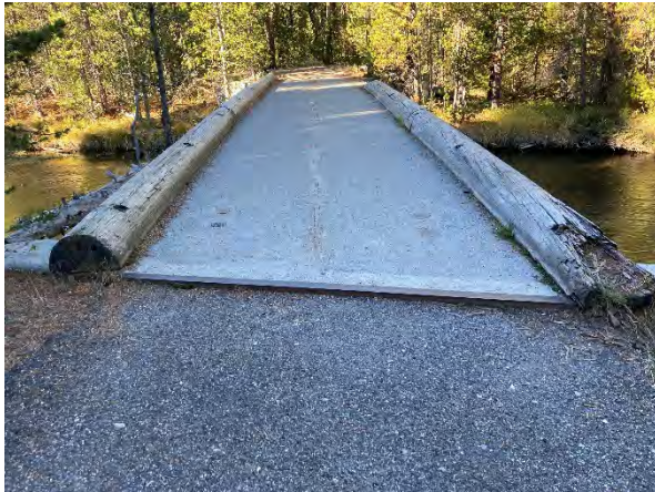
Transition between trail and bridge at Spring Creek
