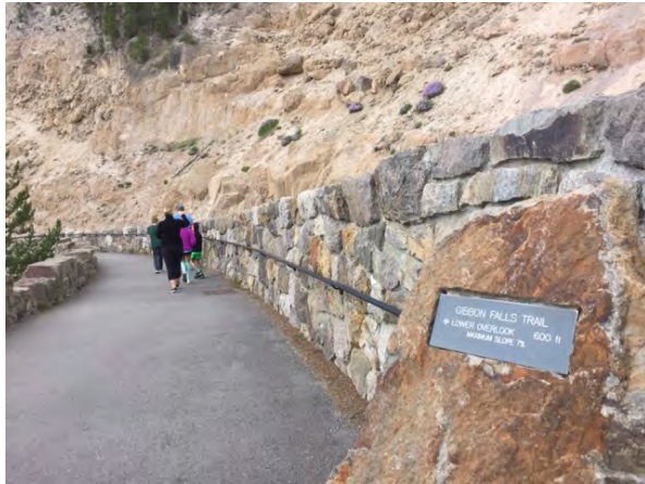
Walkway with railing leading to Gibbon Falls
