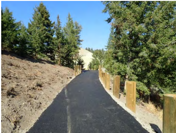
Trail to overlook under construction 2021
