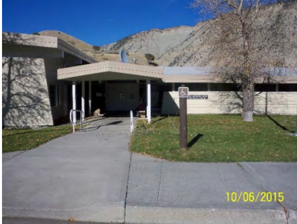
Entrance to Mammoth Community Center (MCC)
