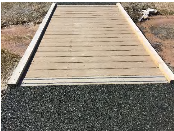
New pavement at the Upper Geyser Basin
