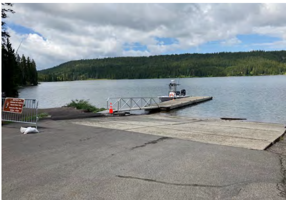
Boat launch, gangway, and dock
