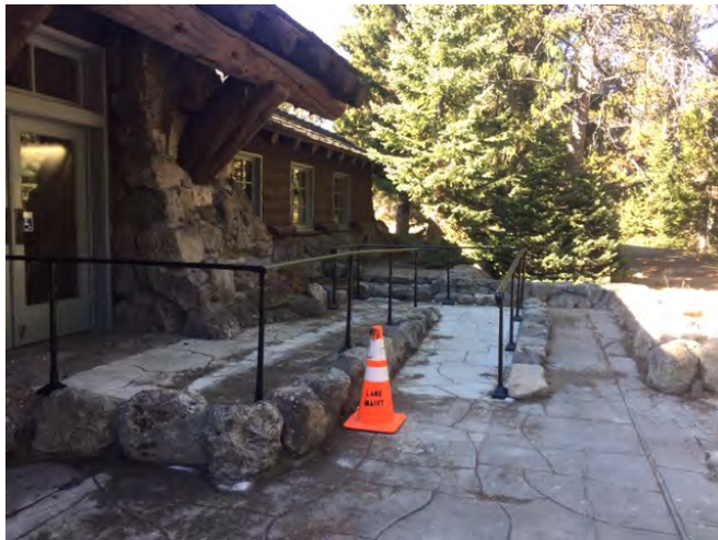
Fishing Bridge Visitor Center entrance ramp
