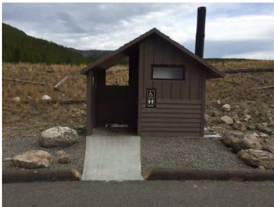
Gibbon Picnic Area vault toilet
