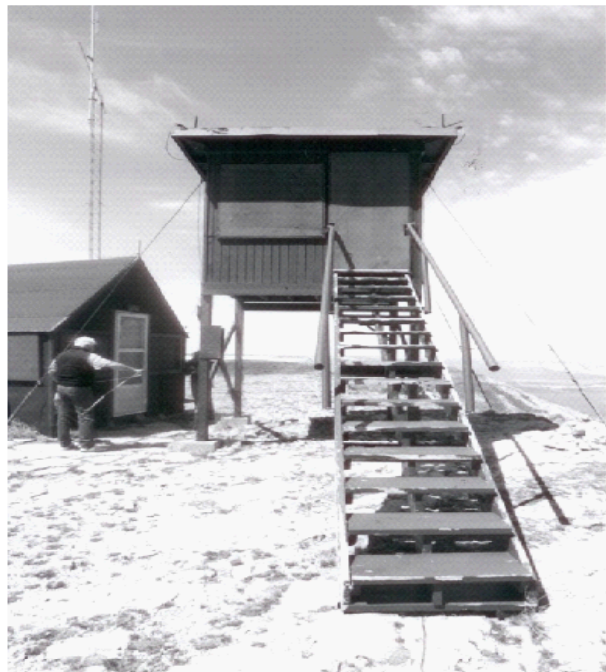
Original fire tower constructed in the mid-1950s. NPS Photo
