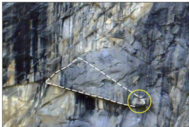
Figure 6. Photograph taken at 07:30 PST on 26 August 2009, following the first rock fall of the sequence (see area 1a in Figure 5). Comparison with high-resolution photographs taken prior to the rock fall (Figure 1(C)) highlights a small (5 m 3 ) failure (yellow circle) located at the tip of a triangular-shaped overhanging slab, a likely point of stress concentration. Subsequent failures later that day resulted in failure of the triangular slab (white dashed line). This figure is available in colour online at wileyonlinelibrary.com/journal/espl
