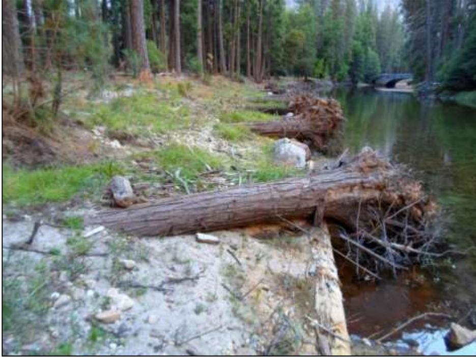
**Figure 5.3.** View downstream from the upper end of Project 5-4, one year after initial construction. Stoneman Bridge in the far distance, with the riprap to be replaced by Project 5-3 also visible just upstream.
