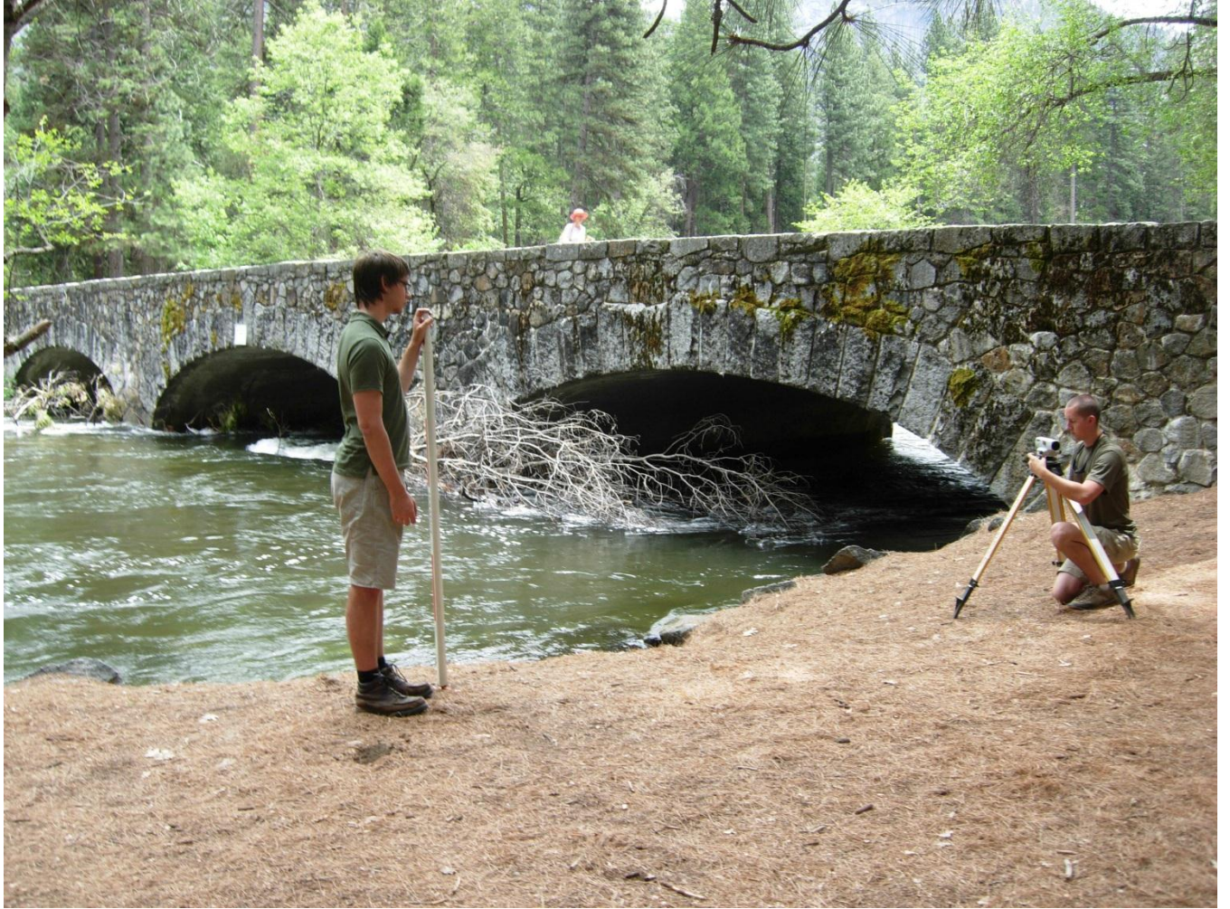
Figure 14. Photograph of water stage measurements during WY2010 showing wood accumulation at Ahwahnee Bridge during WY2010 snowmelt runoff. Photograph taken by YNP personnel, 6/4/2010. Flow is left to right.
