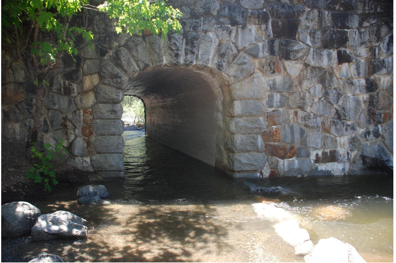
Figure 7. Photograph of flow through river right equestrian tunnel at Clark's Bridge, taken looking upstream. Figures 13 and 14 show the main bridge spans for Clark's and Ahwahnee Bridges. Photograph taken by YNP personnel, 6/7/2010.
