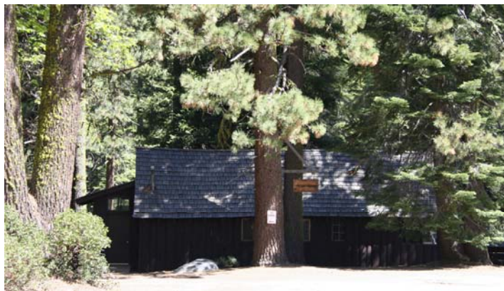
Figure 2-2. Building on Heavily Forested Campus at Crane Flat
