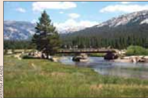
Footbridge near Parsons Lodge (Segment 3)
