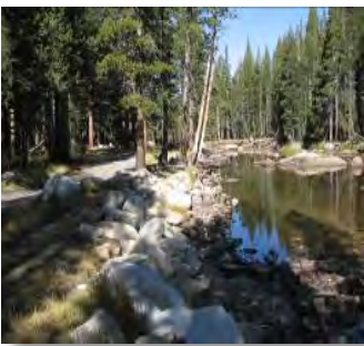
Fig. 1-27. Riprap along river in Tuolumne Campground
