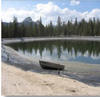
Fig. 1-29. Sewage Treatment Pond
