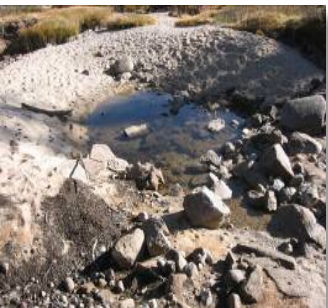
Fig. 1-18. Ponding below culvert at Budd Creek
