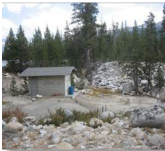
Fig. 1-30. Pump station associated with treatment pond
