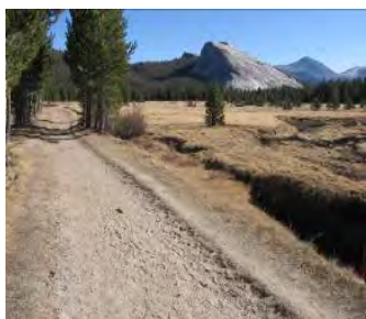
Fig. 1-24. Headcut and ditch adjacent to trail
