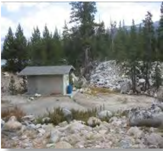
Fig. 1-30. Pump station associated with treatment pond
