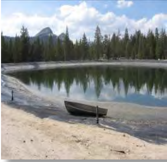
Fig. 1-29. Sewage Treatment Pond
