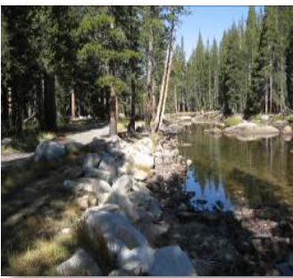
Fig. 1-27. Riprap along river in Tuolumne Campground
