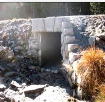
Fig. 1-19. Budd Creek culvert
