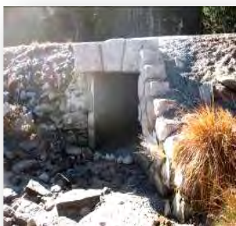
Fig. 1-19. Budd Creek culvert
