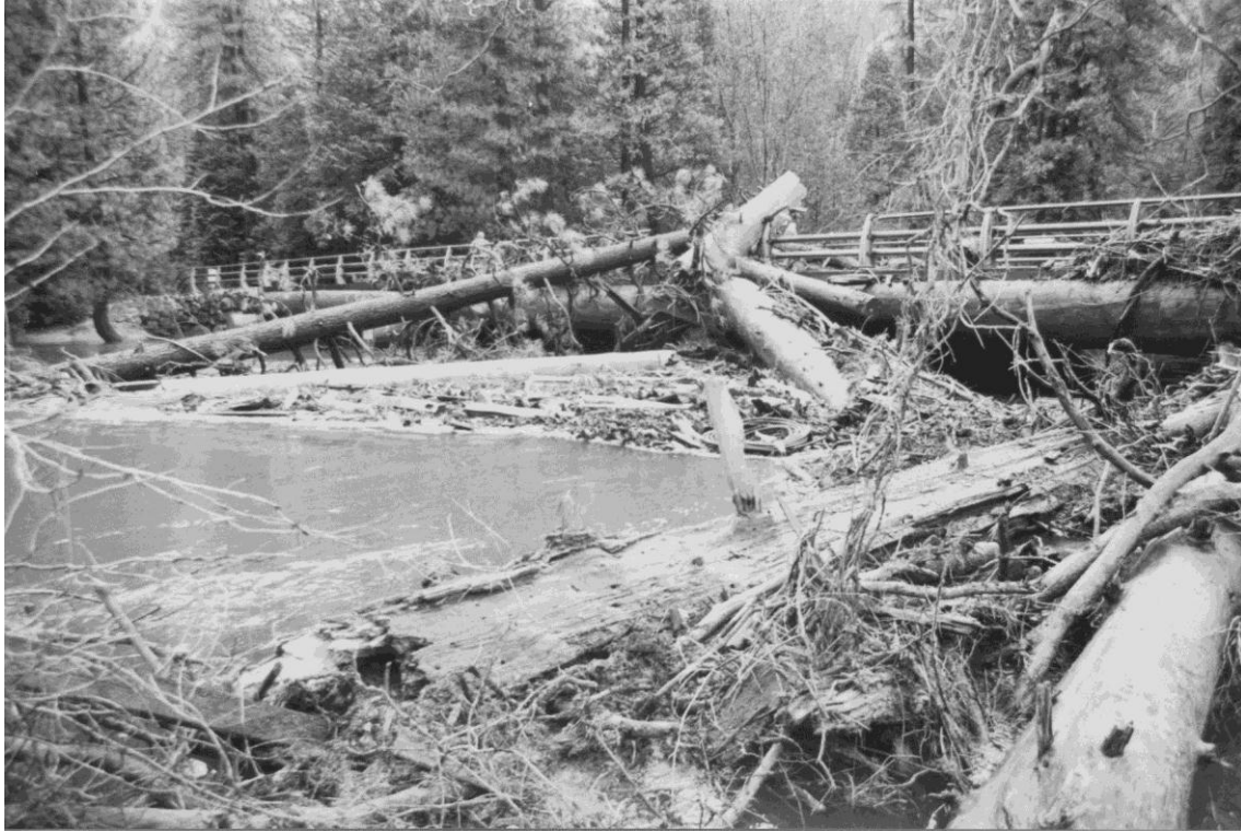
Figure 18. Photograph of large wood accumulated on El Capitan Crossover Bridge immediately following the 1997 flood. The large wood blocks most of the river right 1/3 side of the bridge. Photograph is taken from the river right bank looking downstream towards the bridge. Photograph taken by YNP personnel in January 1997; photograph courtesy of the Yosemite National Park Research Archive.
