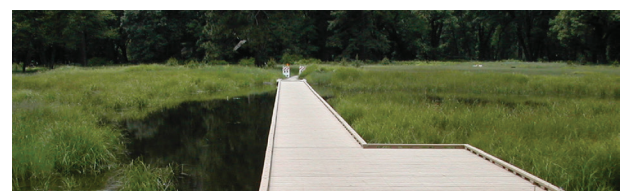
Raised boardwalks, like this one through Cook's Meadow, provide access through wet meadows while maintaining the natural meadow connectivity and hydrologic flow.
