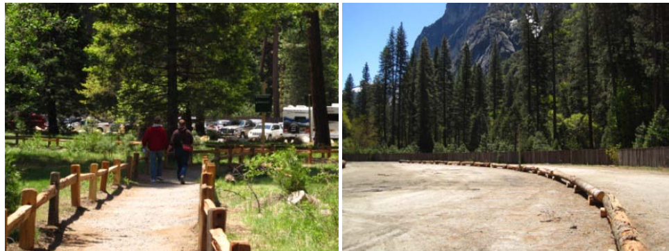
Figure13: Post and rail fencing (Left) and log and block fencing (right).
