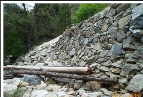
Dry Stack Wall at Failing Section (Concrete Barrier)
