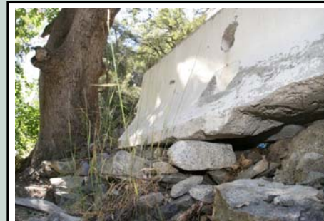
Undercut Concrete Barrier at Failing Section
