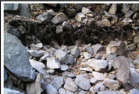
Undercut at Failing Section
