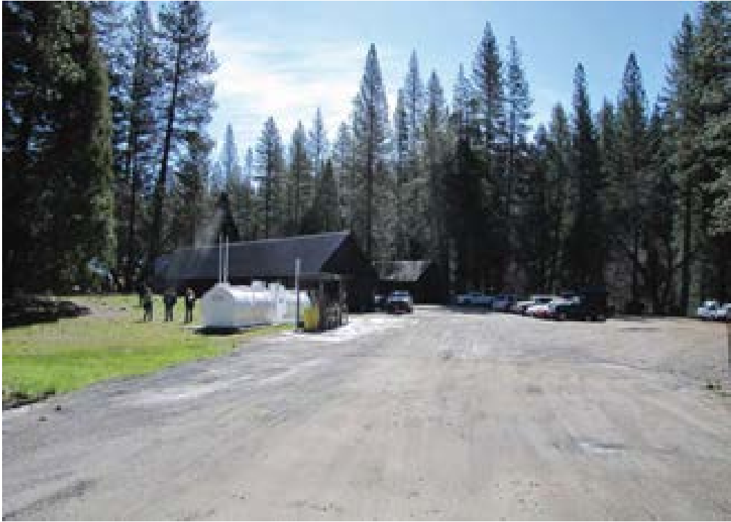
Figure J-32: Wawona CCC-Era Buildings, Ineligible (Draft CLI)
