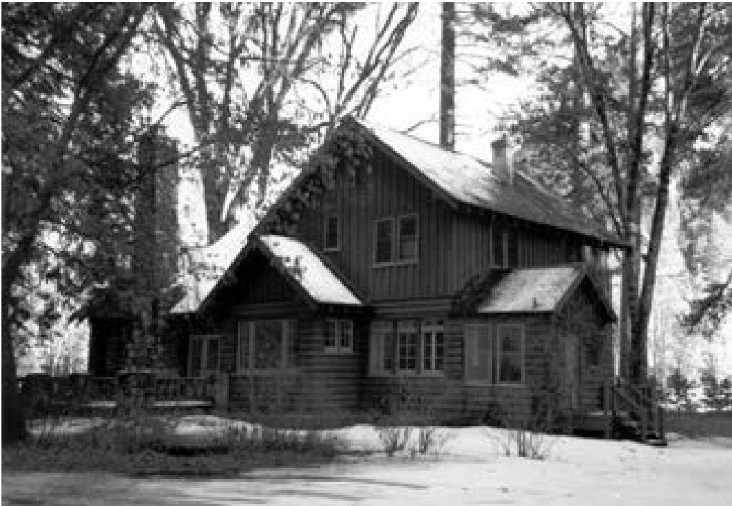
Figure J-21: Superintendent's House (Residence 1), Yosemite Village Historic District/Yosemite Valley Historic District
