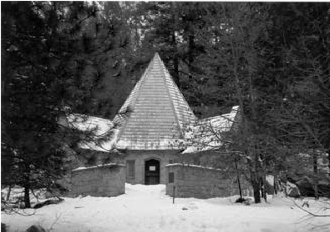
Figure J-15: Le Conte Memorial Lodge, National Historic Landmark/Historic Structure/ Yosemite Valley Historic District
