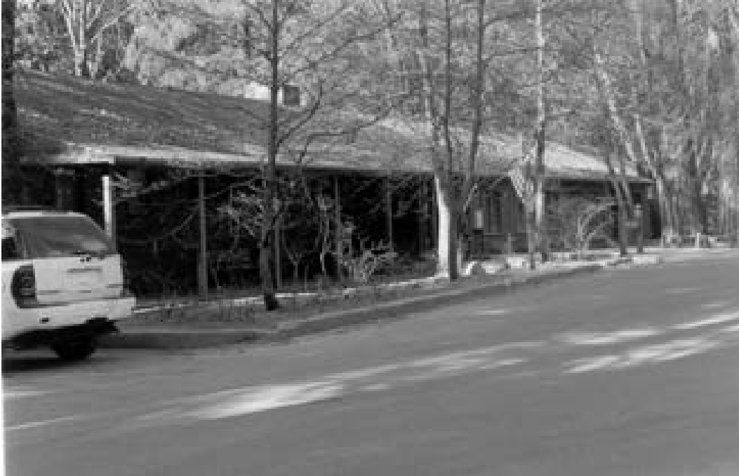
Figure J-18: Concessioner Headquarters Building (Yosemite Village), Yosemite Valley Historic District
