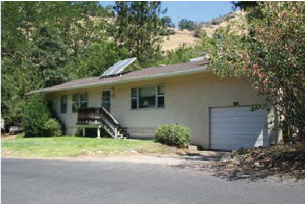
Figure J-30: Rancheria Flat Mission 66-Era Housing (Rancheria, El Portal), Not Evaluated
