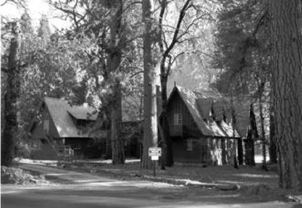
Figure J-20: Ranger's Club National Historic Landmark/Yosemite Village Historic District/Yosemite Valley Historic District
