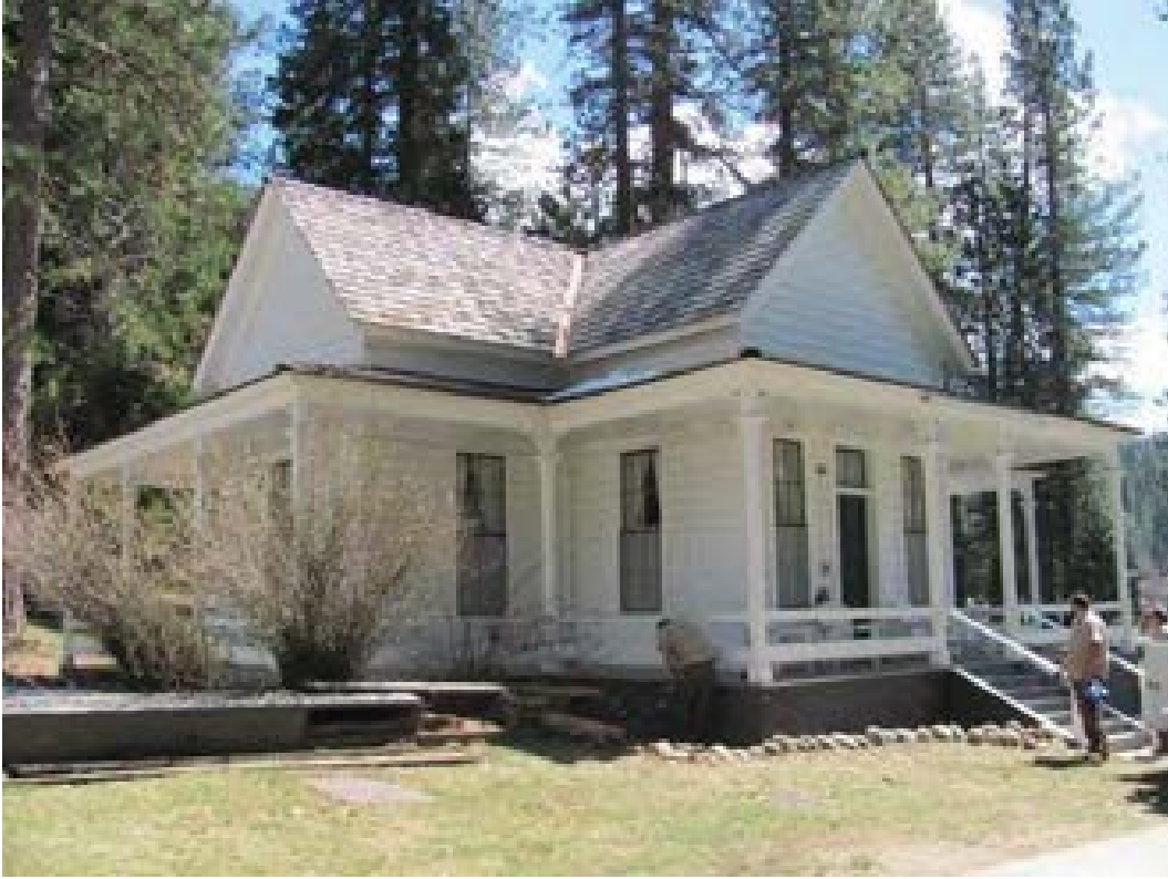
Figure J-36: Manager's Cottage (Little White), Wawona Hotel National Historic Landmark/Historic District
