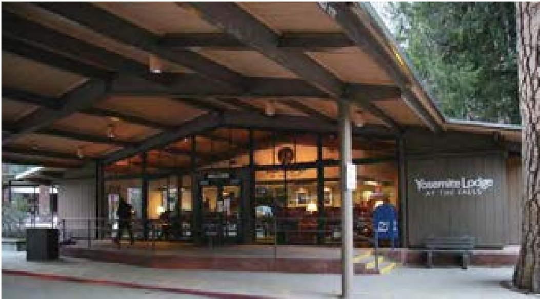
Figure J-22: Yosemite Lodge Registration Building, Yosemite Lodge, Not Evaluated
