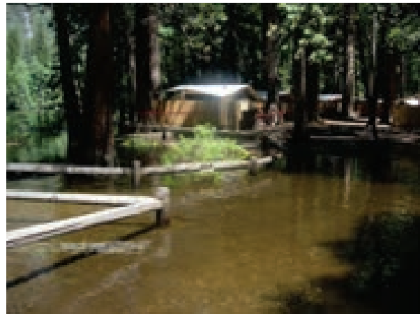
Figure 11: Frequently flooded area at housekeeping camp.
