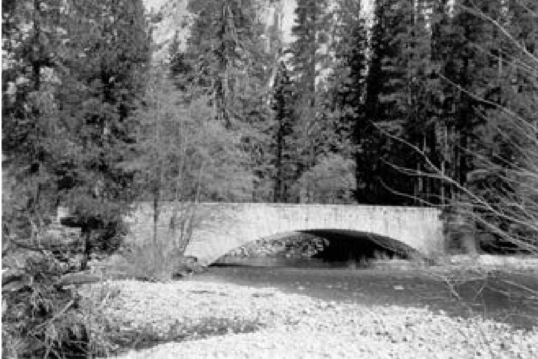
Figure J-2: Sugar Pine Bridge, Yosemite Valley Bridges Historic District/ Yosemite Valley Historic District
