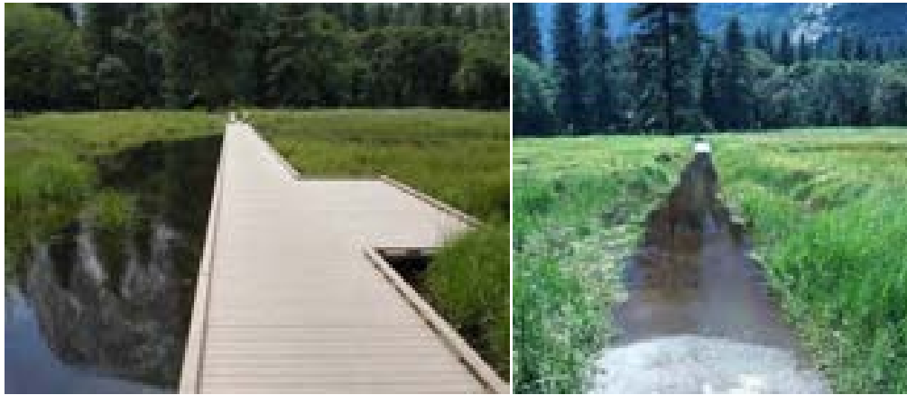
Figure 17: Trails through frequently inundated wet meadows, such as in cook's meadow pre-restoration (left), cause periperal vegetation trampling and soil compaction and make access difficult. A boardwalk installed in 2005 allows for visitor access into the meadow environment and protects the meadow soils and hydrology.
