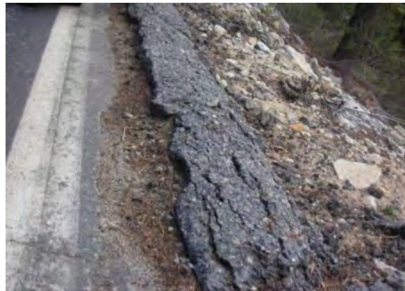
FIGURE 4. FAILED CURB
