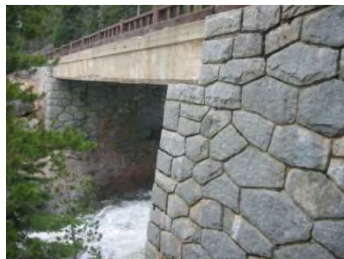
FIGURE 19. SOUTH FORK TUOLUMNE RIVER BRIDGE
