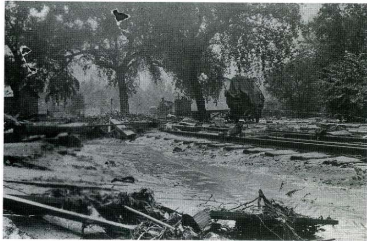
Looking east at the results of the August 13, 1913 cloudburst and flood from the vicinity of the present Standard Oil Co. plant in El Portal. Jim Law collection
