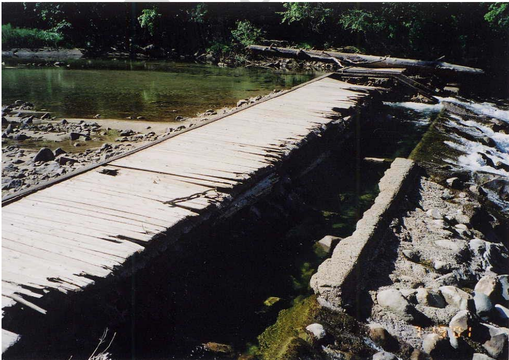
Photo 2.4-14. Before Dam Removal (from North Bank) – 2001 (NPS 2001)
