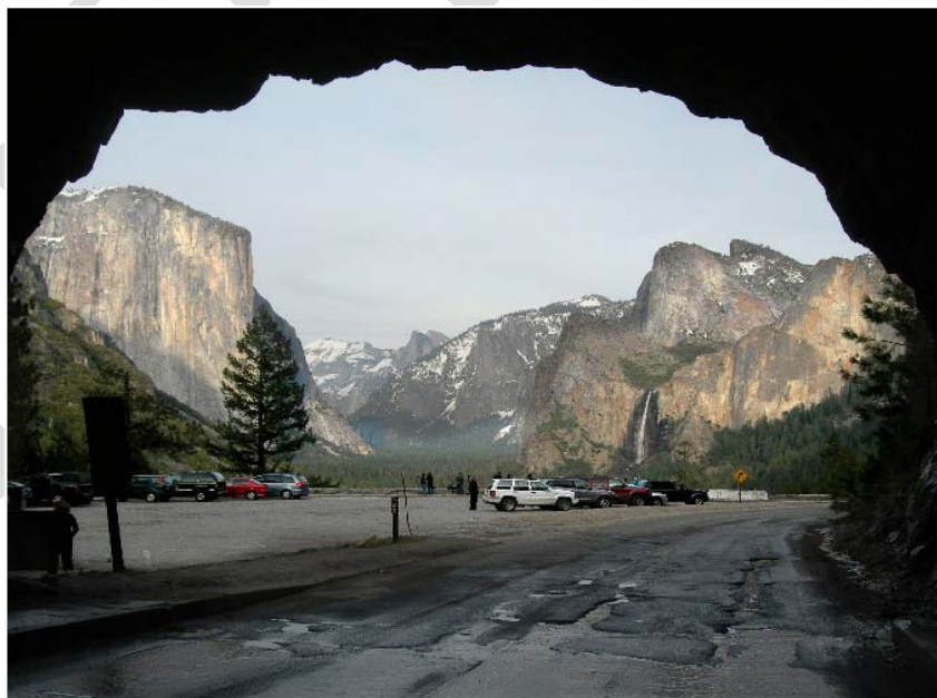
Photo 2.4-11. Wawona Road Tunnel View (Following the Tunnel View Rehabilitation Project) – undated (NPS 2009)
