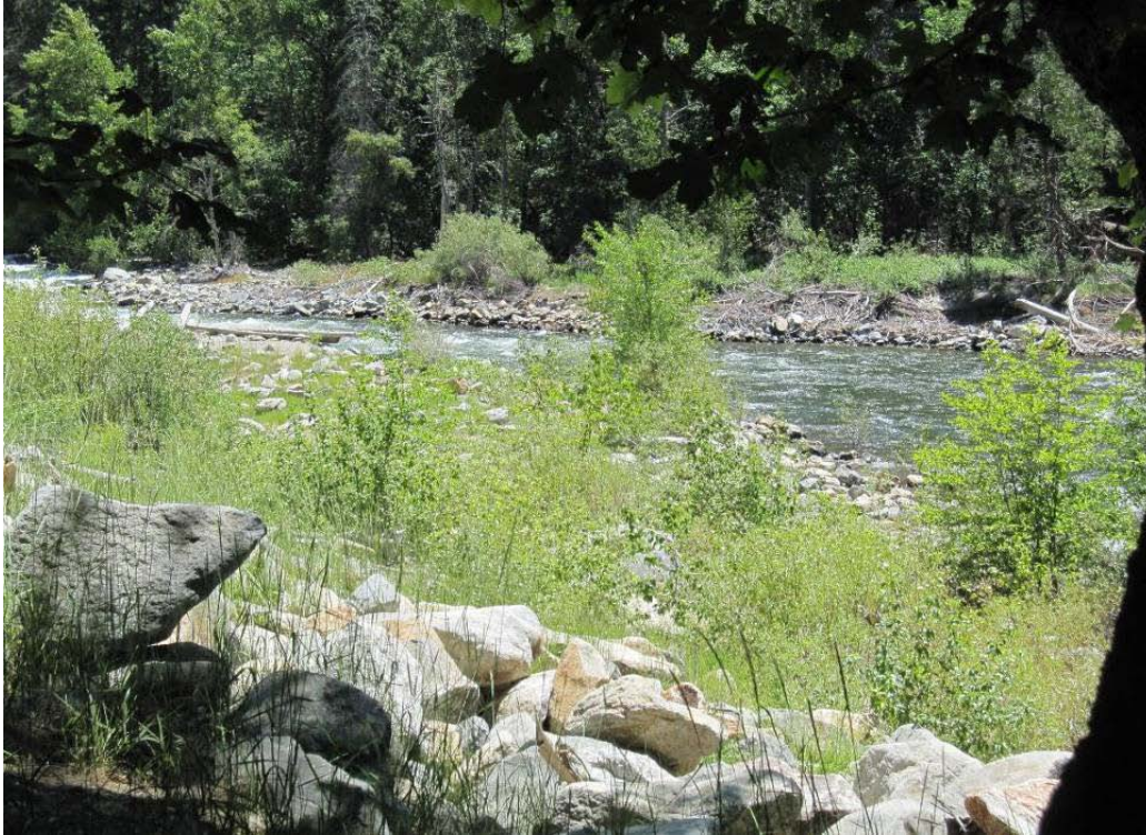
Photo 2.4-15. After Dam Removal (from North Bank) – 2010 (ESA 2010)
