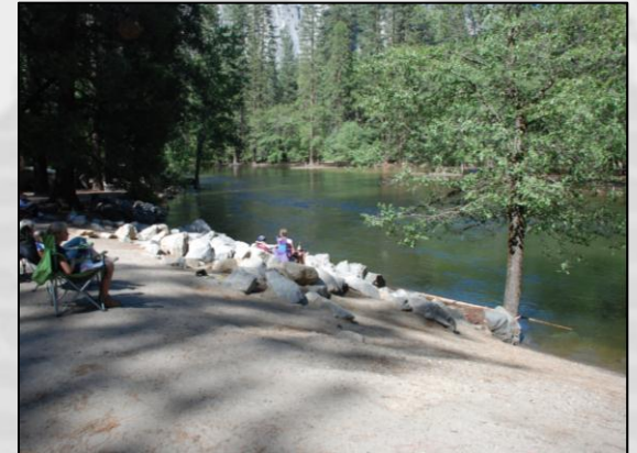
Denuded and riprapped riverbank
