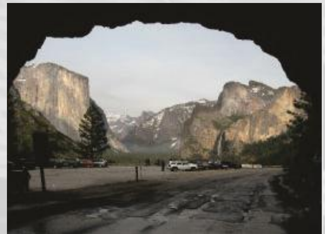
After Tunnel View Restoration , 2008
