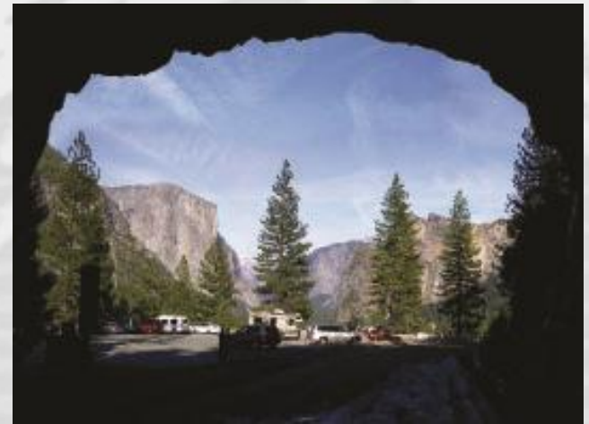
Before Tunnel View Restoration , 2007
