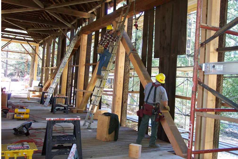
Photo 2.5-2: Wawona Covered Bridge 2005 (NPS 2005)
