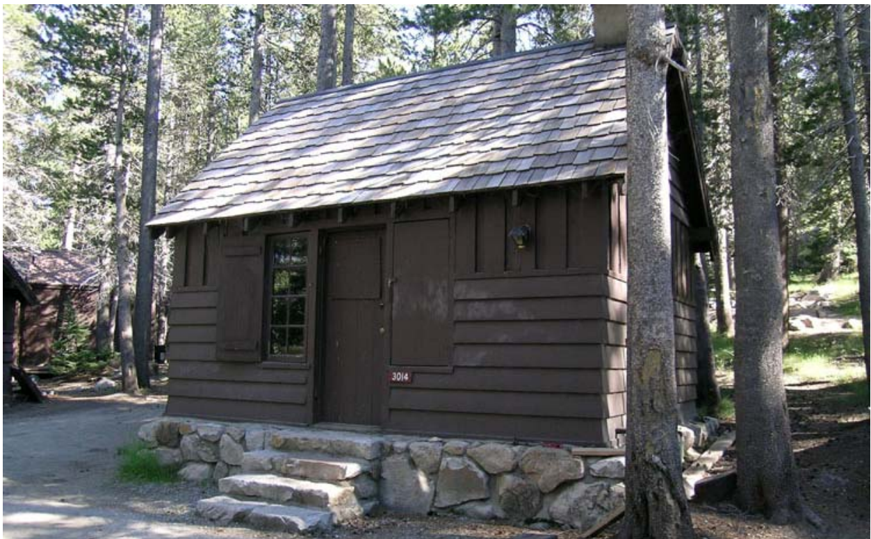
Buildings and Structures #21: CCC-constructed bunkhouse (bldg. #3014). (YOSE, 2006)
