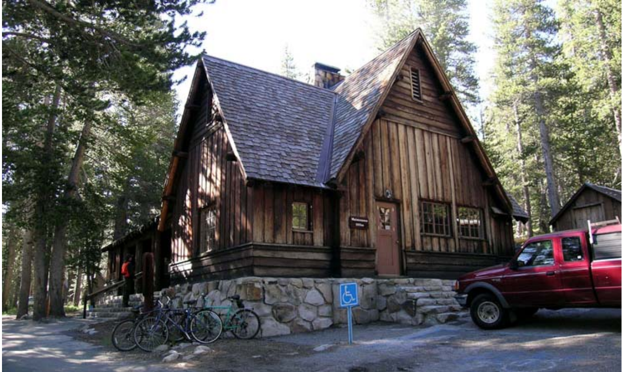
Buildings and Structures #20: CCC-constructed Mess Hall (bldg. #3014), now Tuolumne Meadows Visitor Center. (YOSE, 2006)
