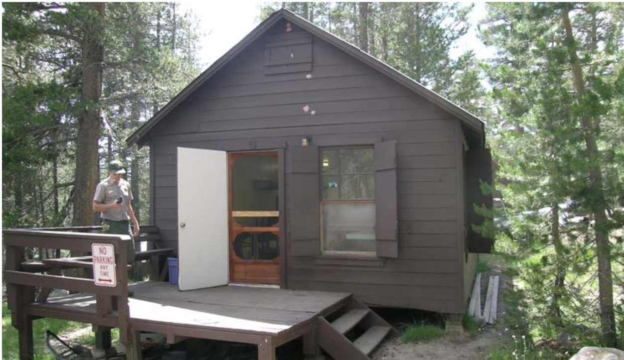
Buildings and Structures #10: View of the mess hall (bldg. #3083), facing west, located at the Insect Research Station. (YOSE, 2006)
