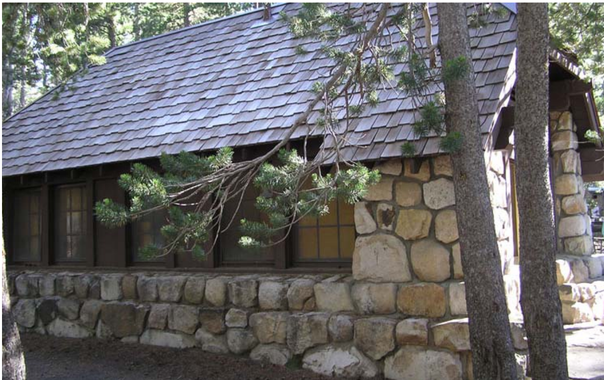
Buildings and Structures #14: View of a 1934 rustic comfort station (bldg. #3022), located at the Tuolumne Meadows Public Campground. (YOSE, 2006)
