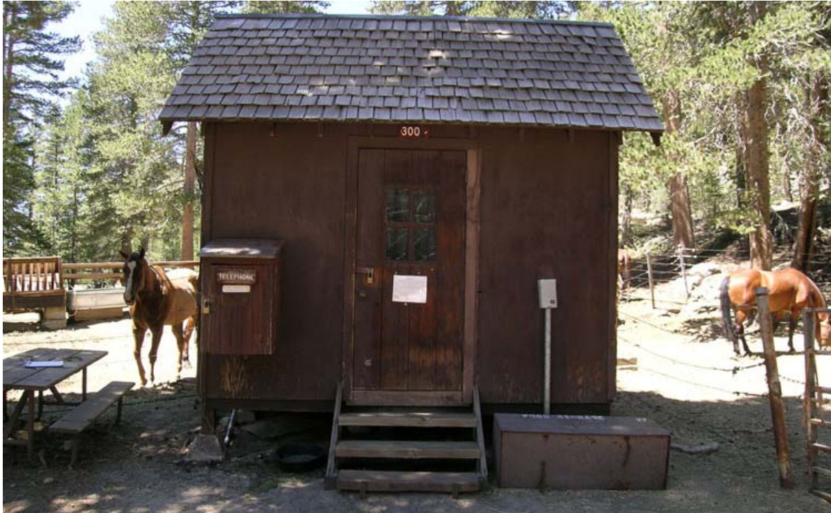
Buildings and Structures #6: View of the pack shed (bldg. #3004) and telephone box, facing northwest, in the Administrative Area. (YOSE, 2006)
