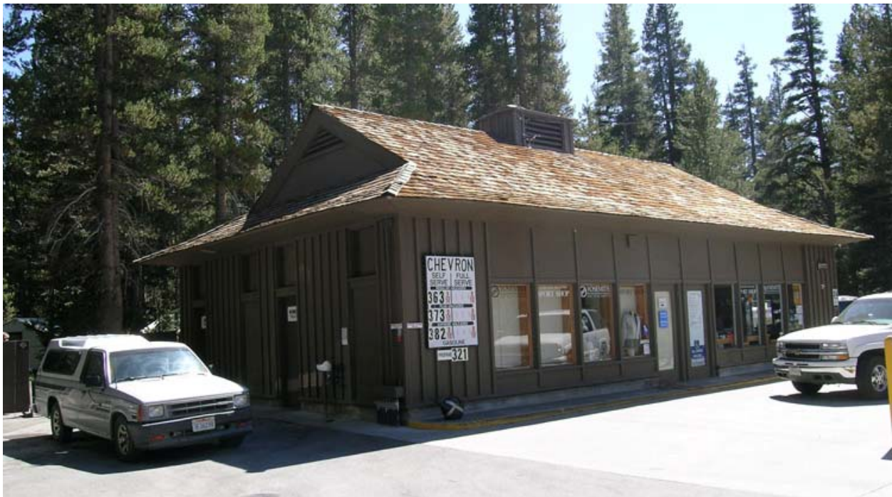
Buildings and Structures #19: View of the Tuolumne Meadows Gas Station, facing southwest. (YOSE, 2006)
