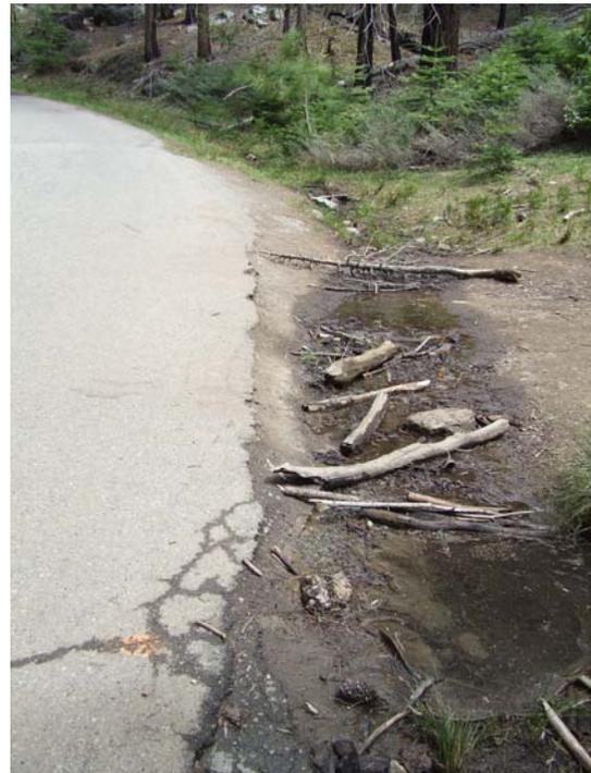
Figure 3-16 – Drainage Channel along the Mariposa Grove Road within the Grove
