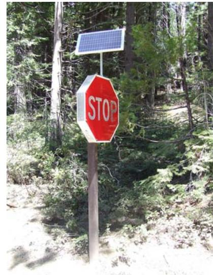
**Figure 3-38 – Solar-powered Sign at South Entrance**
