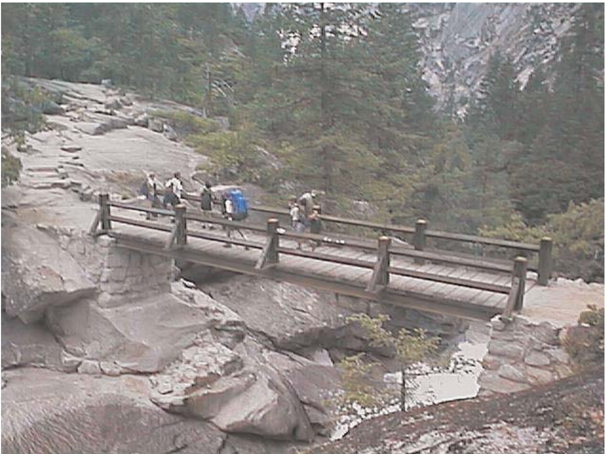
An "after" shot of the repaired Silver Apron Bridge
