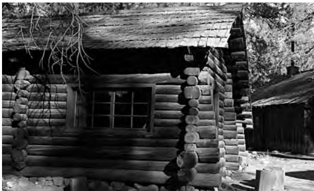
TOP Grey Barn, Pioneer Yosemite History Center (2008) GH MIDDLE Wells Fargo Building, Pioneer Yosemite History Center (2007) GH BOTTOM Log structure, Pioneer Yosemite History Center (2007) GH
