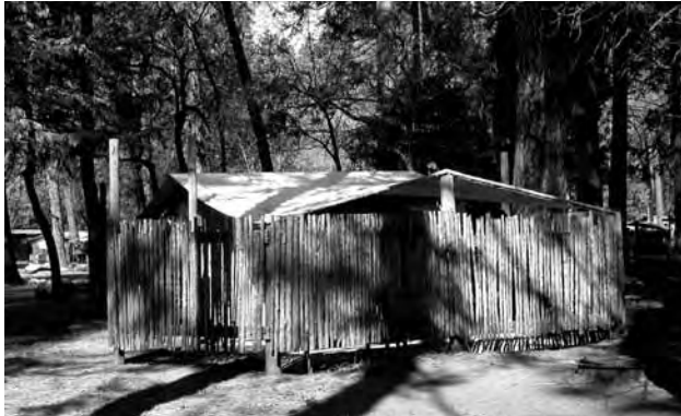
TOP Cabin on the river, Housekeeping Camp (2004) GH BOTTOM Cabin with privacy screen, Housekeeping Camp (2004) GH
