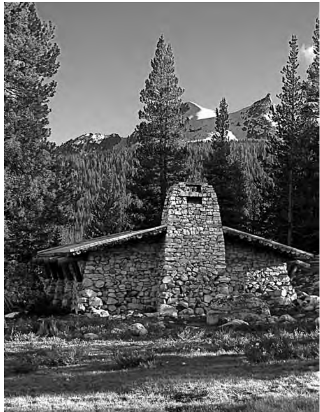
North elevation, Parsons Memorial Lodge (2010) RF
