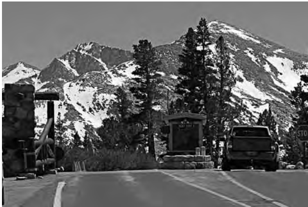
TOP Comfort station, Tioga Pass Entrance Station (2007) GH BOTTOM Tioga Pass Entrance Station (2008) GH
