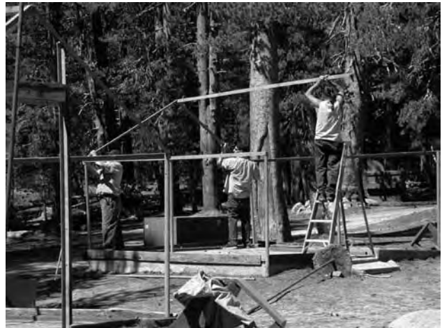
Framing for tent cabins, White Wolf Lodge (2008) GH
