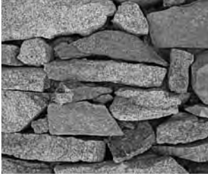
Dry-stack masonry, Vogelsang High Sierra Camp (2007) RF
