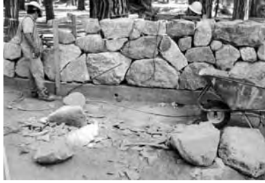
Stone wall under construction at Lower Yosemite Fall area (2004) RF
