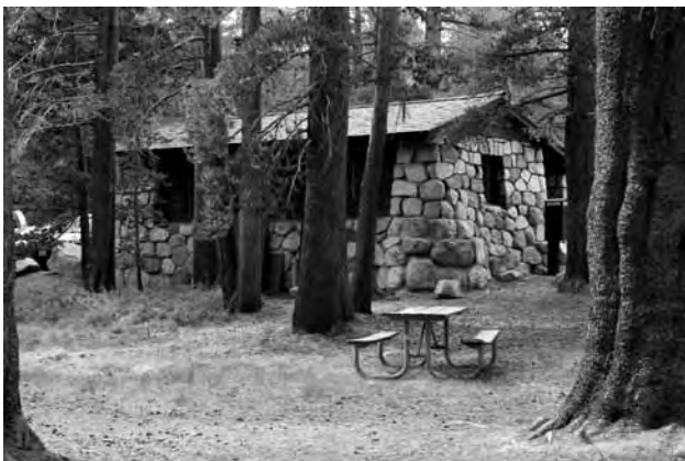
Campground Reservation Building, Tuolumne Meadows (2008) GH
