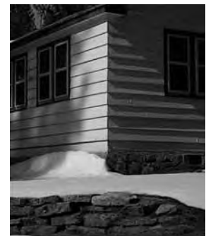
Masonry detail, Wawona Ranger Office (2008) GH
