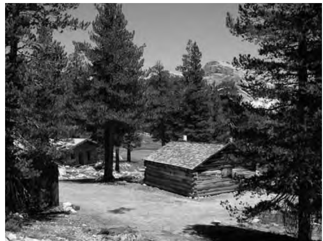
Parsons Memorial Lodge and McCauley Cabin (2007) GH
