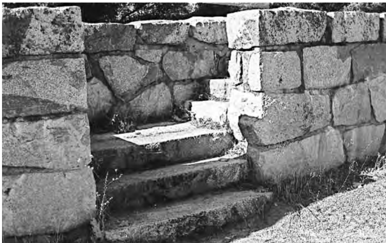
Recessed steps and retaining wall, Tunnel View, Wawona Road (2009) TP
