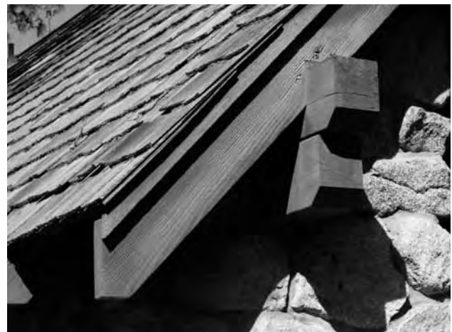
Roof detail, comfort station, Tuolumne Meadows Campground (2008) GH
