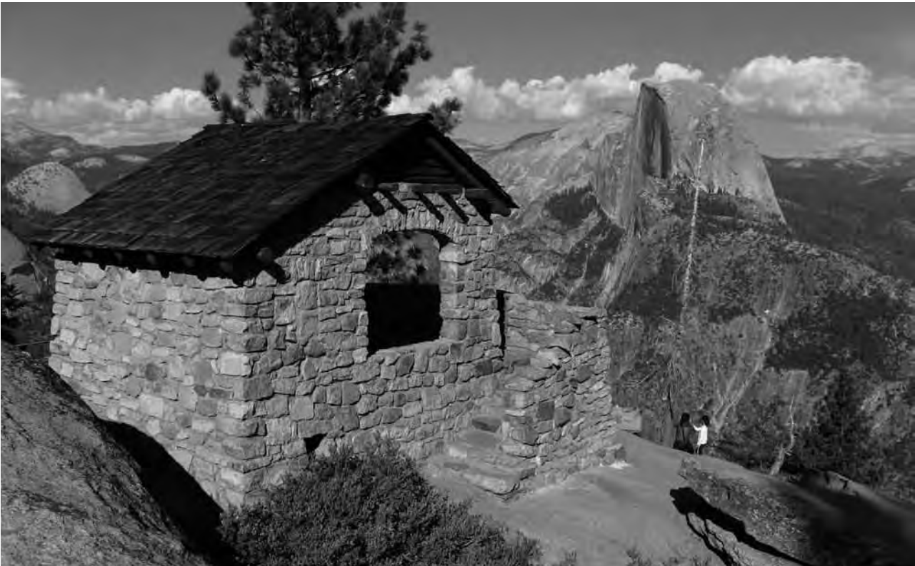
Geology Hut, with masonry showing incised steps into granite, Glacier Point (2008) RF
