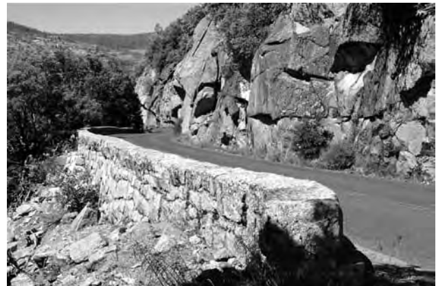
Site-sourced, worked-granite guard walls, Hetch Hetchy Road (2008) GH
