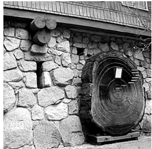
Lower masonry wall of Museum, Yosemite Village (2004) GH
