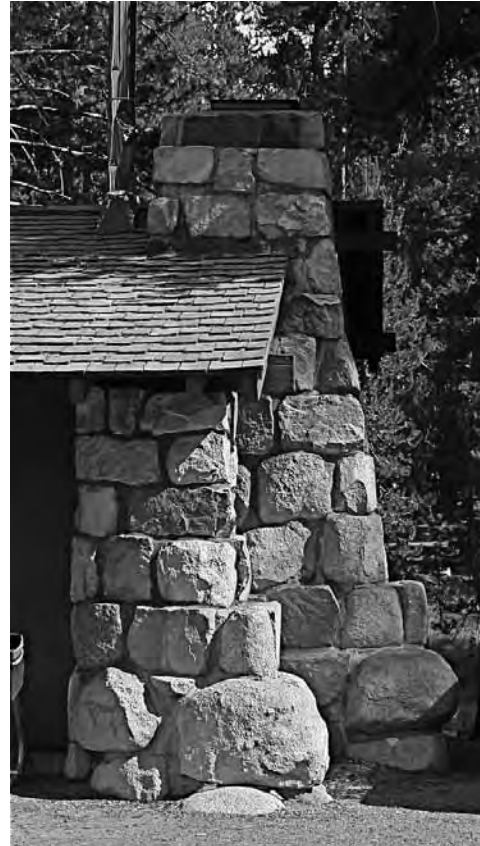
Porch and chimney detail, Campground Reservation Building, Tuolumne Meadows (2008) GH
