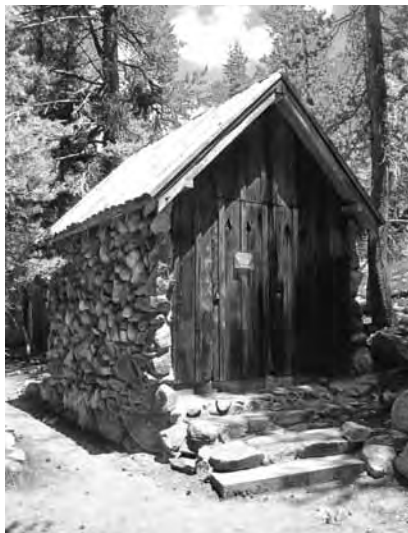
Storage shed, Glen Aulin High Sierra Camp (2004) RF
