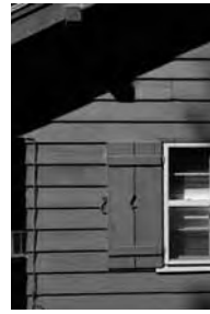
Detail, ranger residence, South Entrance (2008) GH
