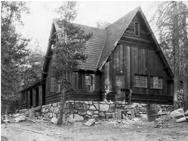
CCC Mess Hall, Road Crew Camp (date unknown) YRL
