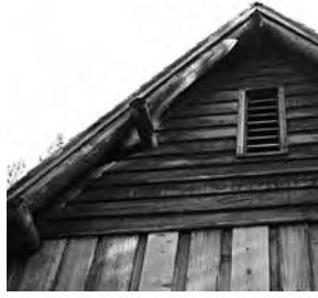
LEFT Exterior wall of Administration Building, Yosemite Village (2004) GH RIGHT Roof framing and wall treatment, CCC Mess Hall, Tuolumne Meadows (2007) GH
