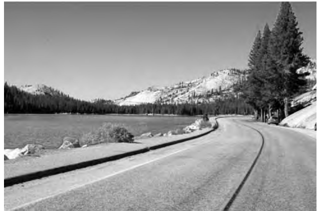
Tioga Road at Tenaya Lake (2008) GH
