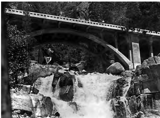
TOP Fitted riprap, Big Oak Flat Road (2008) GH MIDDLE Half Dome View, Big Oak Flat Road (2010) DN BOTTOM Concrete bridge over Cascade Creek, Big Oak Flat Road (date unknown) YRL-RA
