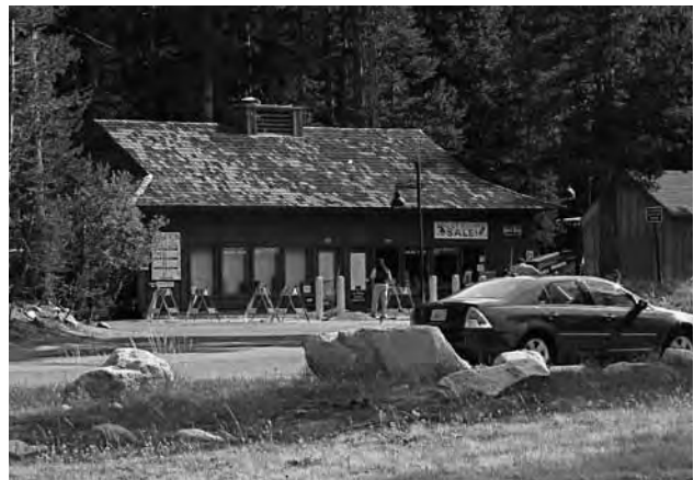
TOP Tuolumne Meadows Store and Grill (2008) GH MIDDLE Canvas roof removed for winter, Tuolumne Meadows Store and Grill (2010) RF BOTTOM Tuolumne Meadows Gas Station (2008) GH
