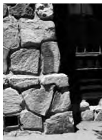
Detail of masonry at CCC Mess Hall, Road Crew Camp (2008) GH
