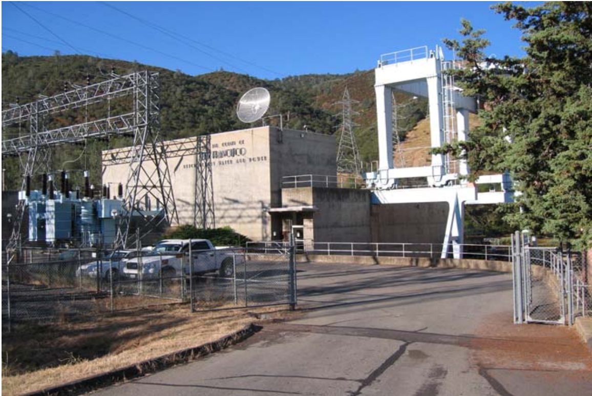
Southeast-facing view of Moccasin Powerhouse Figure 3.10.2-2
