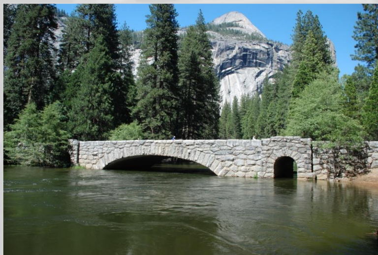
Stoneman Bridge at high water
