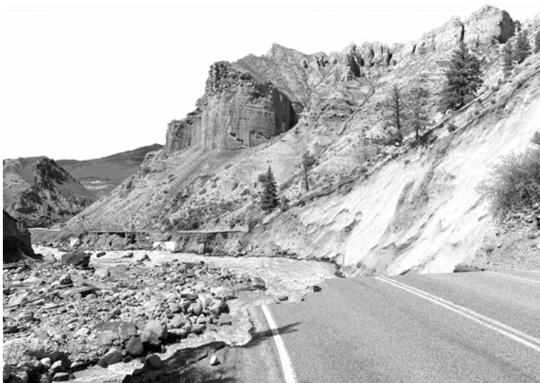
One of many washouts on the North Entrance Road from Gardiner, MT, to Mammoth Hot Springs.
