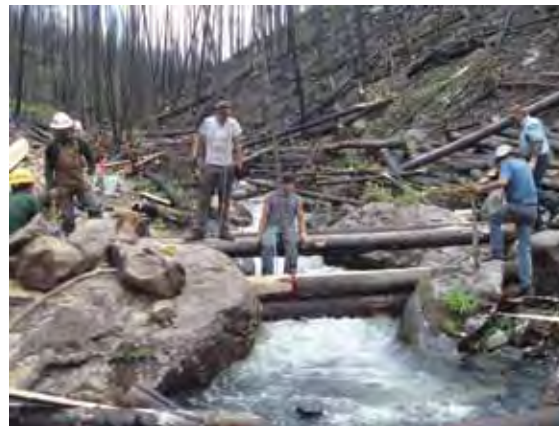
Montana Conservation Crew and contractors place barrier logs.
