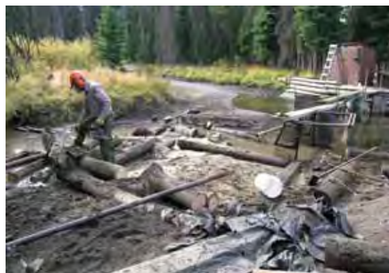
Fisheries technician Brian Ertel and Student Conservation Association interns Kate Olson and Brendan Crowley work to remove a damaged weir from Clear Creek.
