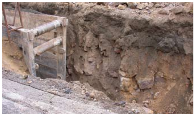
Figure 10. Natural fractures exposed within a sewage trench connecting the water treatment plant with the comfort station at Norris Geyser Basin. The trench exposed fractured (northeast, northwest, north) and hydrothermally altered Lava Creek B tuff.
