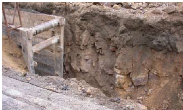
Figure 10. Natural fractures exposed within a sewage trench connecting the water treatment plant with the comfort station at Norris Geyser Basin. The trench exposed fractured (northeast, northwest, north) and hydrothermally altered Lava Creek B tuff.
