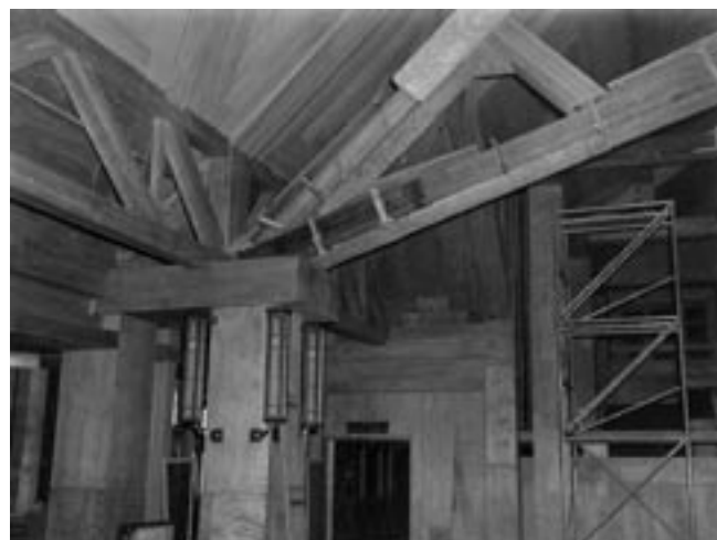
The structural failure in the roof trusses of the Canyon Hotel lobby was caused by foundation problems.
