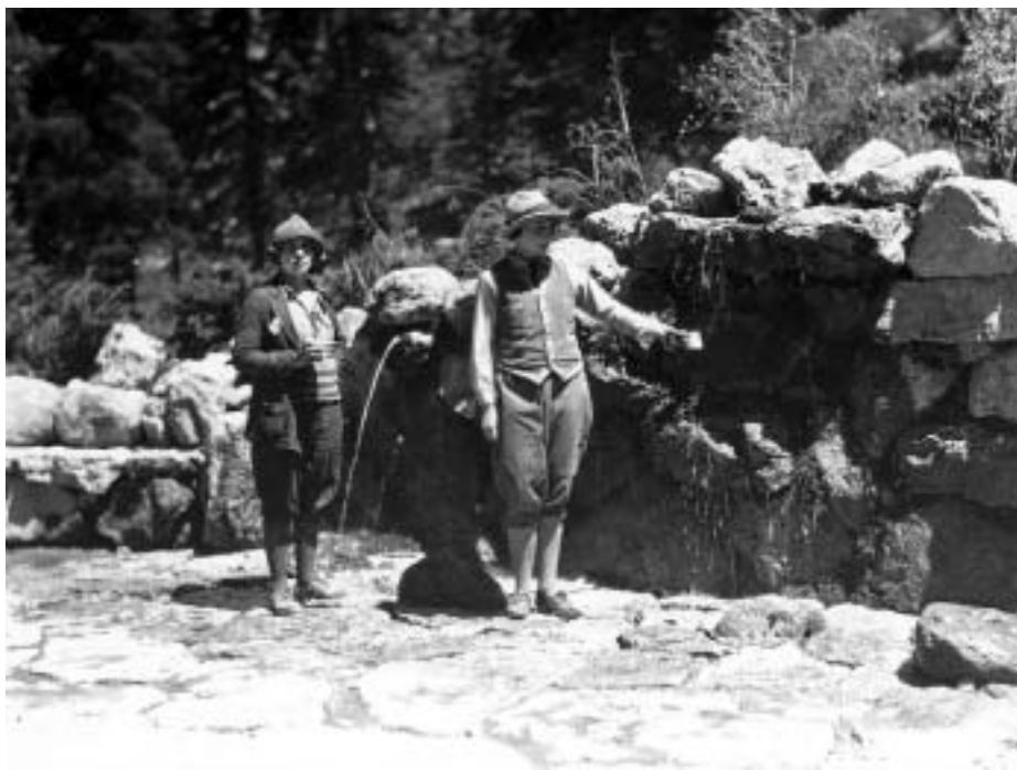
Two women stand on the new flagstone deck of Apollinaris Spring, 1925. Limestone slabs for the deck were mined at the nearby Hoodoos formation.
