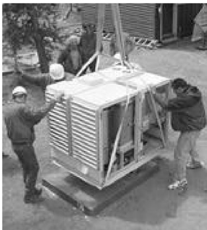
Fuel cell being installed at West Entrance on May 6, 2002. NPS photo.
