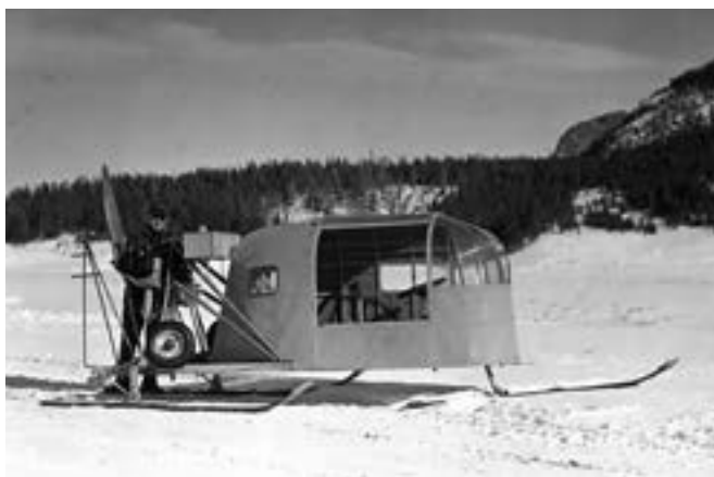
Snowplane on Swan Lake Flat, c. 1945. These winter vehicles consisted of passenger cabs set on skis and blown about (without becoming airborne) with a rear-mounted airplane propeller and engine.
