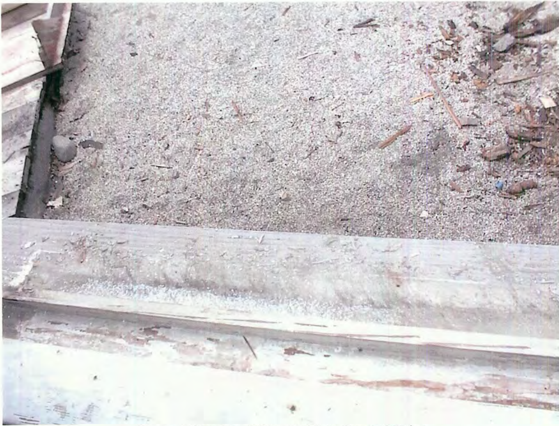
Typical Window Sill with Deteriorated Paint
