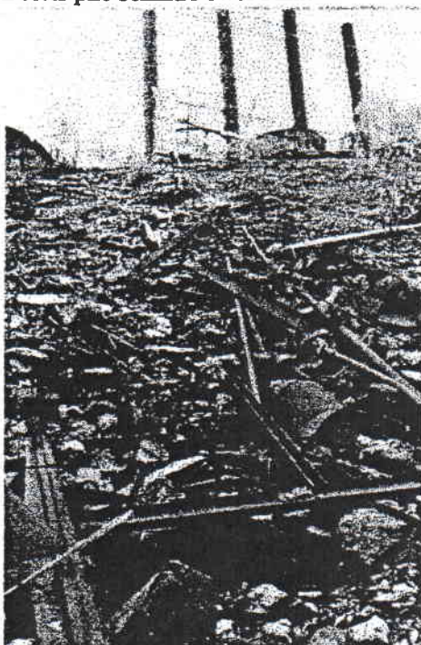
Debris Pile below Power Plant
