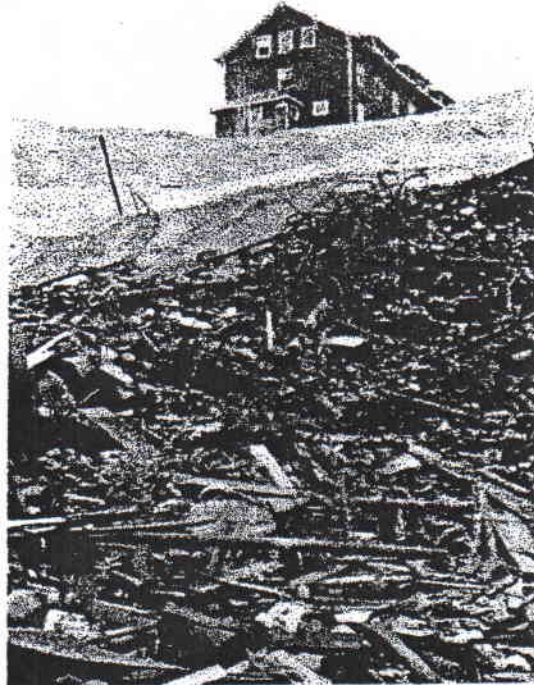
Debris pile below West Bunk house
